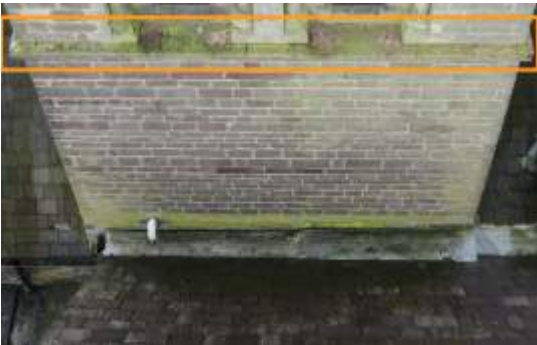
2674745 Severity: 1 Lichen Build Up
