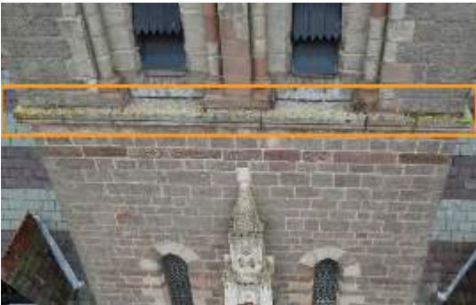
2673981 Severity: 1 Lichen Build Up
