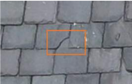
2675498 Severity: 2 Damaged Slate
