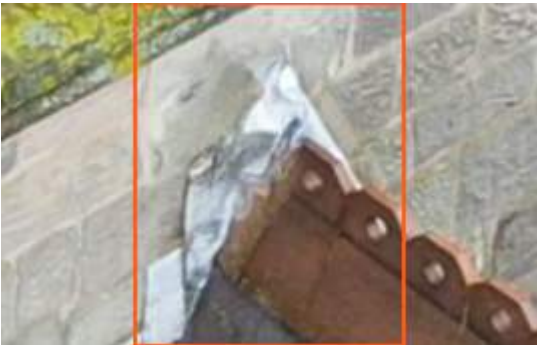
2674002 Severity: 3 Flashing
