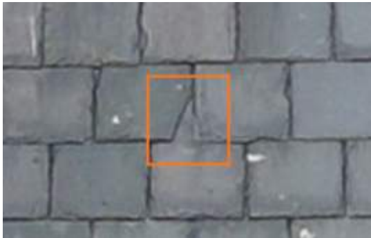
2675533 Severity: 2 Damaged Slate
