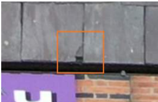
2675841 Severity: 2 Damaged Slate
