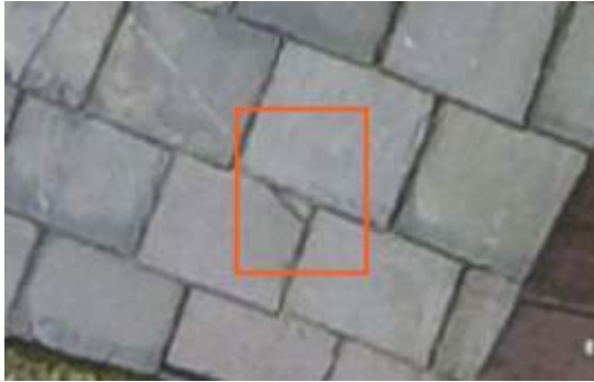
2674732 Severity: 3 Damaged Slate
