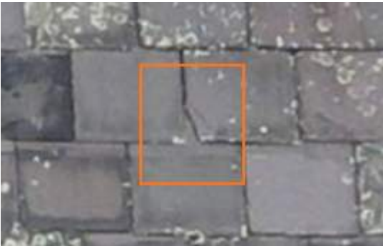
2674763 Severity: 2 Damaged Slate
