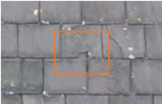
2674782 Severity: 2 Damaged Slate
