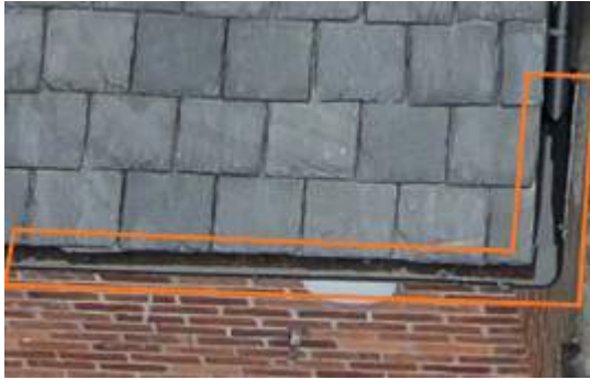
2675505 Severity: 2 Standing Water in Gutter
