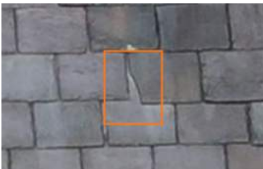
2675546 Severity: 2 Damaged Slate
