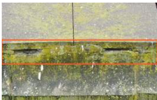
2675859 Severity: 3 Missing Mortar
