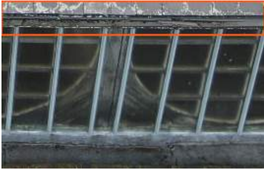
2674781 Severity: 3 Significant Debris in Gutter
