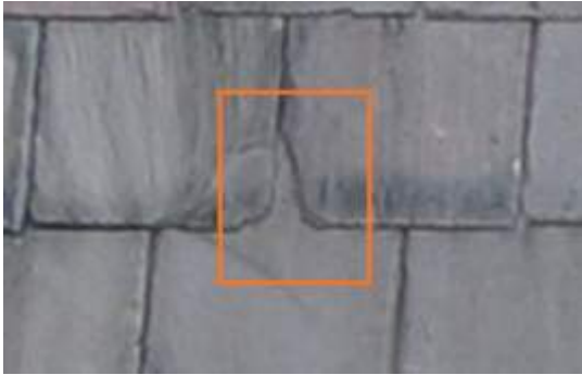
2675764 Severity: 2 Damaged Slate
