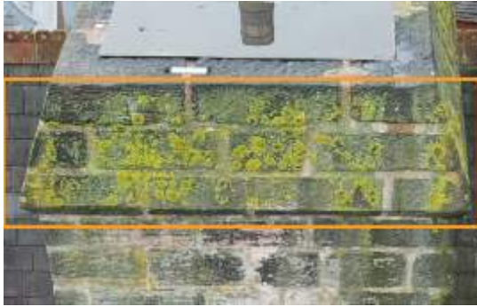
2674537 Severity: 1 Lichen Build Up
