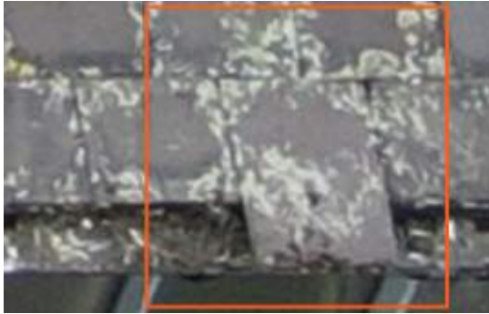
2674771 Severity: 3 Slipped Slate
