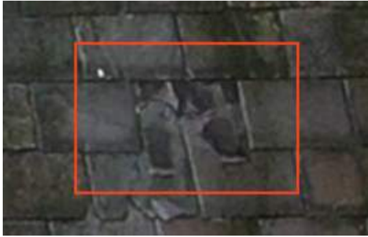
2675550 Severity: 4 Damaged Slate
