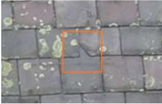
2674789 Severity: 2 Damaged Slate
