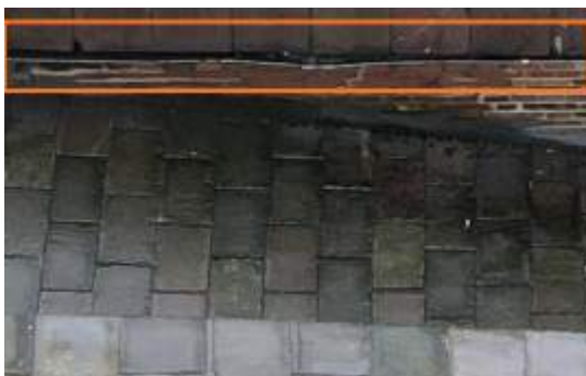
2674642 Severity: 2 Gutter Deformed
