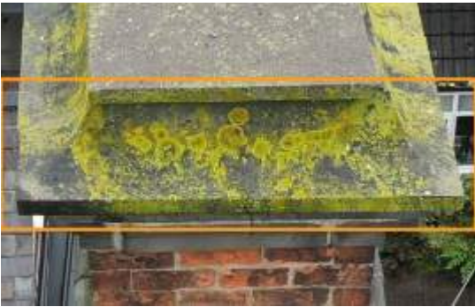
2675894 Severity: 1 Lichen Build Up
