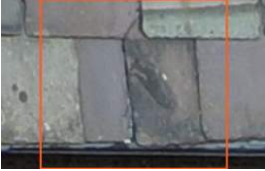
2675804 Severity: 3 Damaged Slate
