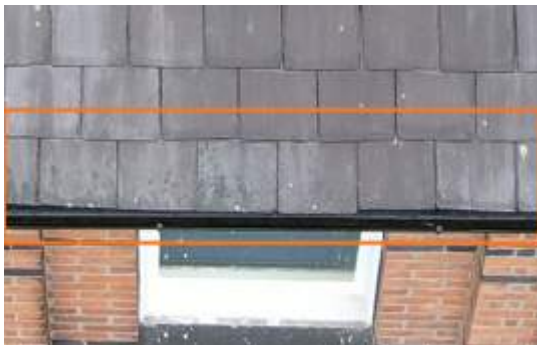
2675836 Severity: 2 Misaligned Slate
