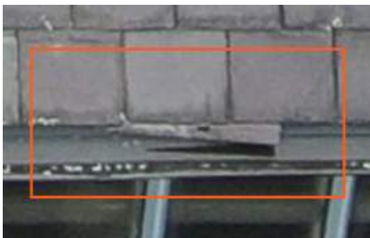
2674788 Severity: 3 Slipped Slate
