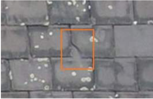
2674764 Severity: 2 Damaged Slate
