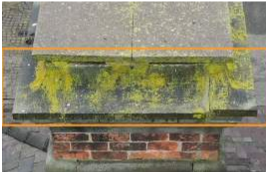
2675889 Severity: 1 Lichen Build Up
