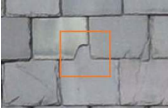
2674833 Severity: 2 Damaged Slate
