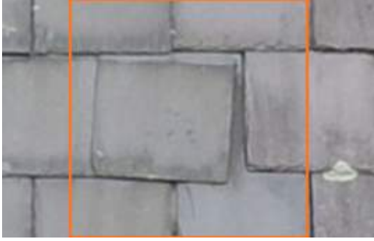
2675783 Severity: 2 Misaligned Slate
