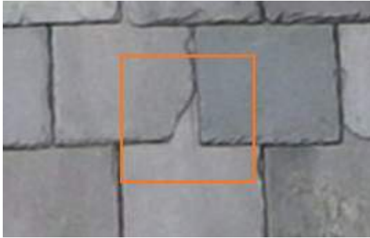
2674826 Severity: 2 Damaged Slate
