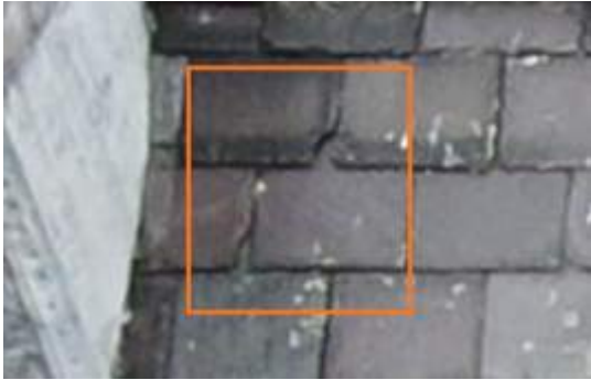
2674766 Severity: 2 Damaged Slate
