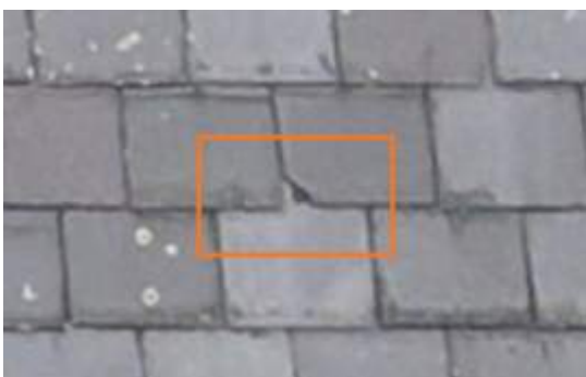
2674784 Severity: 2 Damaged Slate
