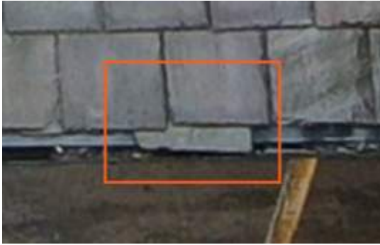
2675537 Severity: 3 Slipped Slate
