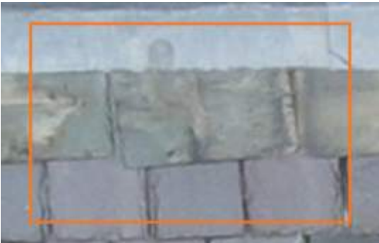
2674841 Severity: 2 Misaligned Slate
