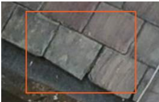
2674588 Severity: 3 Slipped Slate
