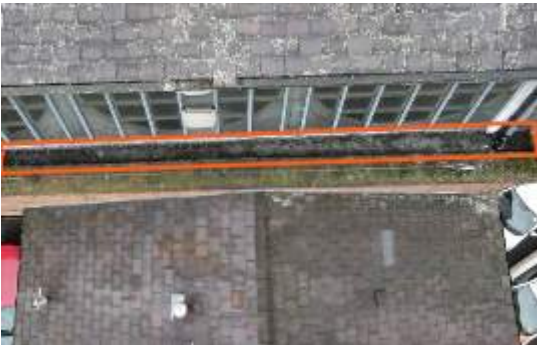
2675909 Severity: 3 Minor Debris in Gutter
