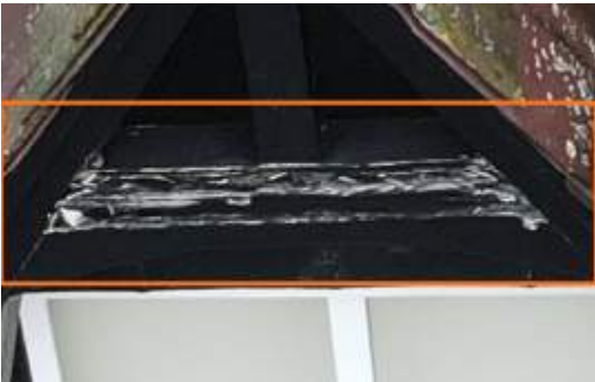
2673959 Severity: 2 Paint Coat Failed
