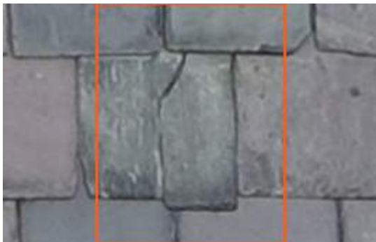
2675794 Severity: 3 Damaged Slate
