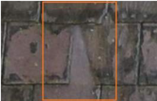
2675768 Severity: 2 Damaged Slate
