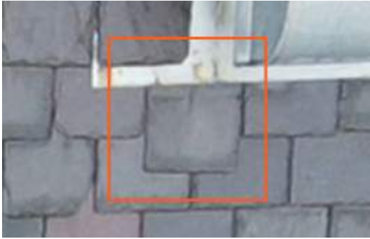
2675480 Severity: 3 Slipped Slate
