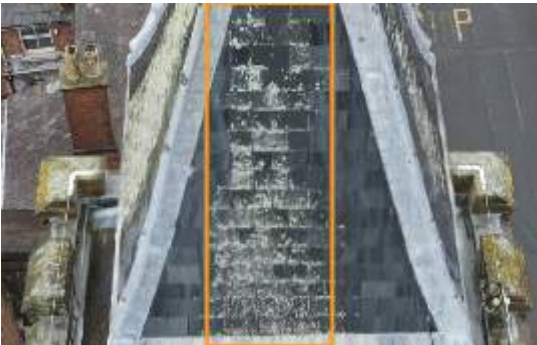
2674750 Severity: 1 Lichen Build Up
