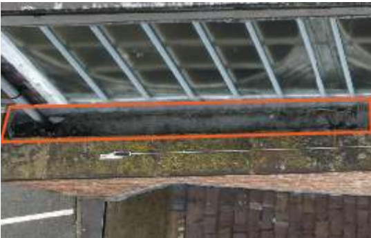
2675910 Severity: 3 Minor Debris in Gutter
