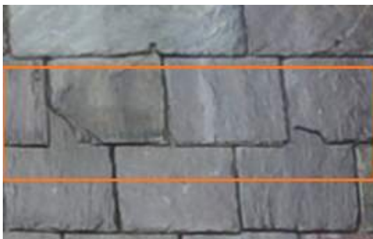
2674819 Severity: 2 Damaged Slate
