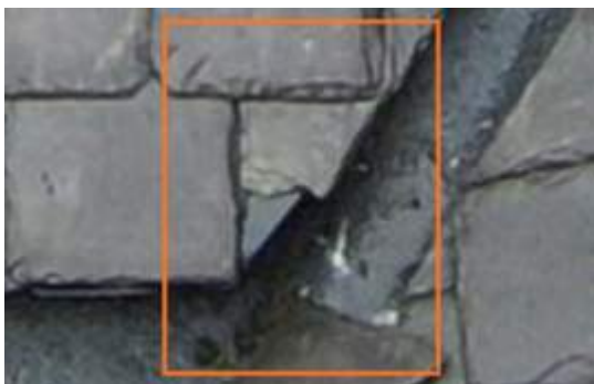
2674828 Severity: 2 Damaged Slate
