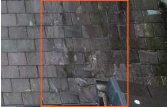
2675565 Severity: 3 Damaged Slate
