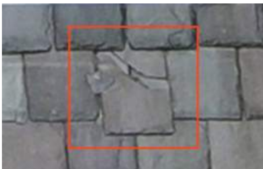
2675536 Severity: 4 Damaged Slate
