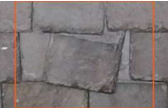
2673672 Severity: 3 Slipped Slate
