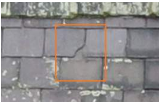
2674755 Severity: 2 Damaged Slate
