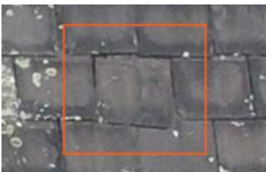
2674769 Severity: 3 Slipped Slate
