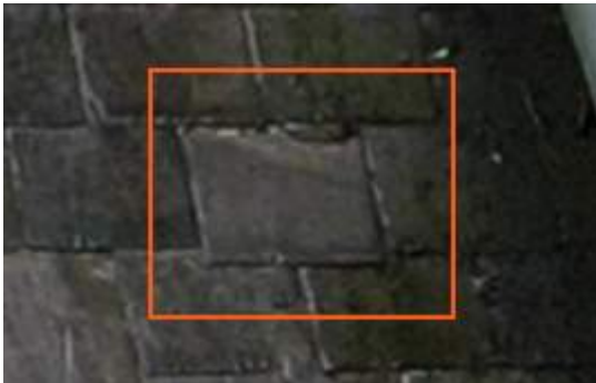
2675566 Severity: 3 Slipped Slate
