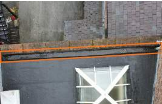
2674742 Severity: 2 Evidence of Standing Water
