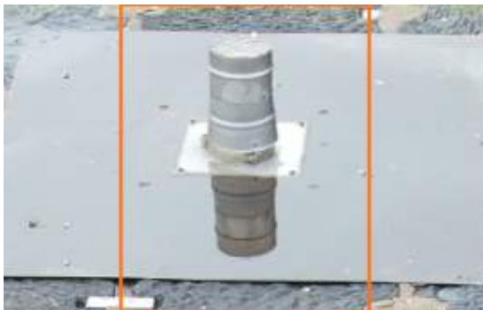
2674335 Severity: 2 Evidence of Standing Water
