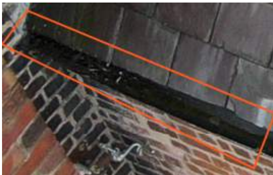
2674327 Severity: 3 Minor Debris in Gutter
