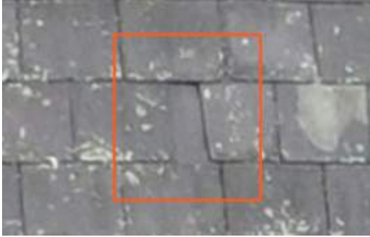
2674756 Severity: 3 Damaged Slate
