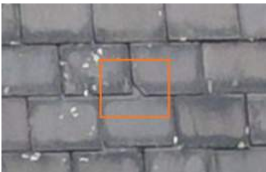
2674768 Severity: 2 Damaged Slate
