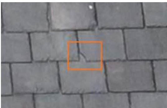
2675543 Severity: 2 Damaged Slate
