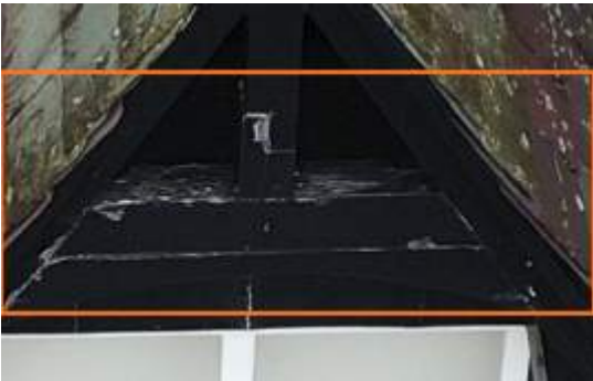
2673973 Severity: 2 Paint Coat Failed
