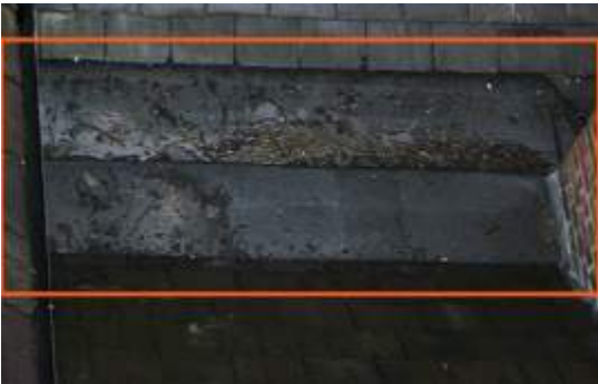
2674309 Severity: 3 Minor Debris in Gutter
