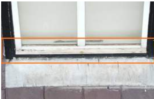
2674253 Severity: 2 Paint Coat Failed
