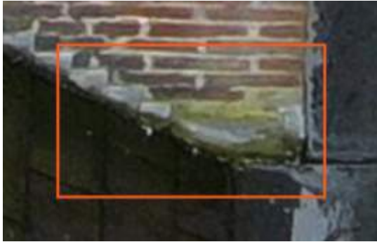
2674554 Severity: 3 Flashing
