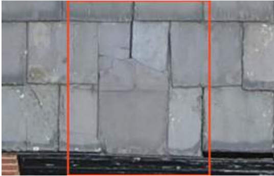
2675739 Severity: 4 Damaged Slate
