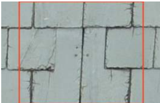
2674188 Severity: 4 Missing Slate
