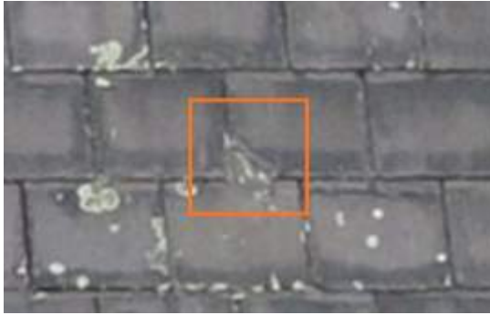
2674770 Severity: 2 Damaged Slate
