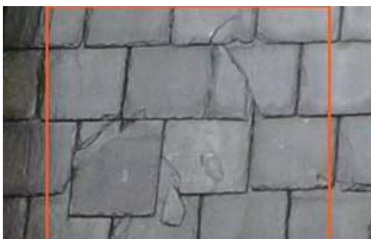
2674830 Severity: 3 Damaged Slate
