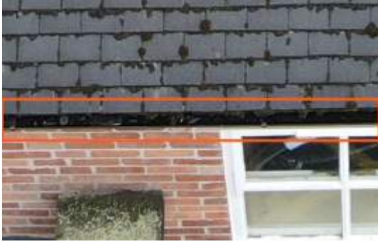
2675681 Severity: 3 Minor Debris in Gutter
