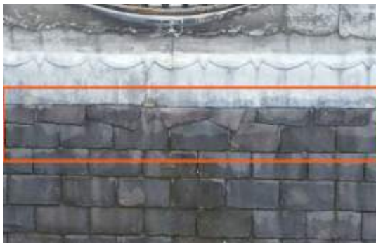
2674748 Severity: 3 Misaligned Slate
