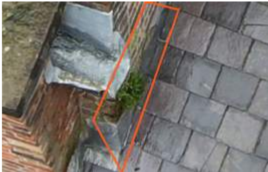
2674733 Severity: 3 Missing Flashing
