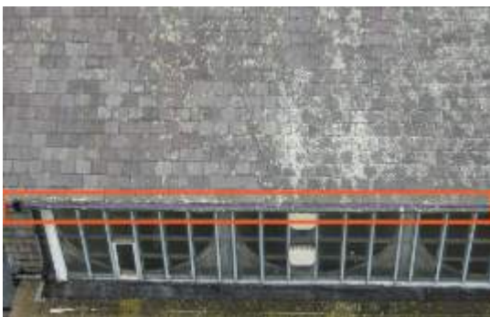
2674759 Severity: 3 Gutter Deformed
