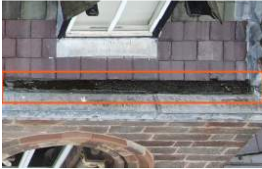
2674214 Severity: 3 Minor Debris in Gutter
