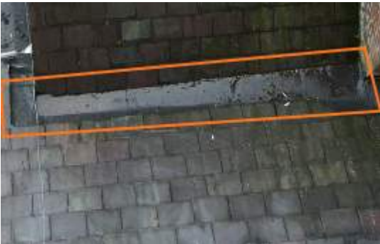
2674587 Severity: 2 Ponding Water
