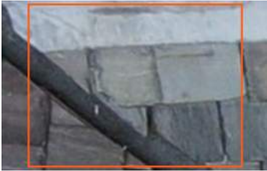
2674844 Severity: 3 Slipped Slate
