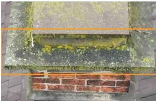
2675868 Severity: 1 Lichen Build Up
