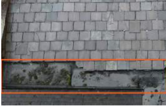
2674831 Severity: 3 Minor Debris in Gutter
