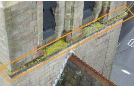
2673831 Severity: 1 Lichen Build Up
