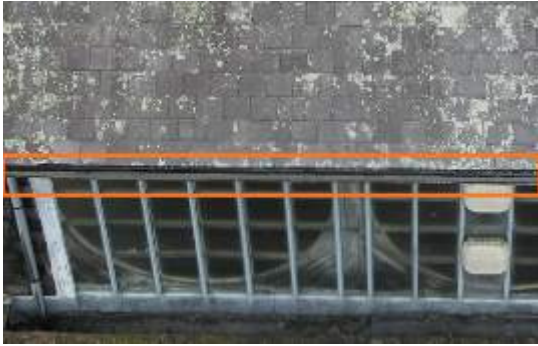
2674780 Severity: 2 Standing Water in Gutter
