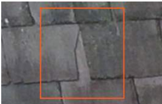
2674288 Severity: 3 Damaged Slate
