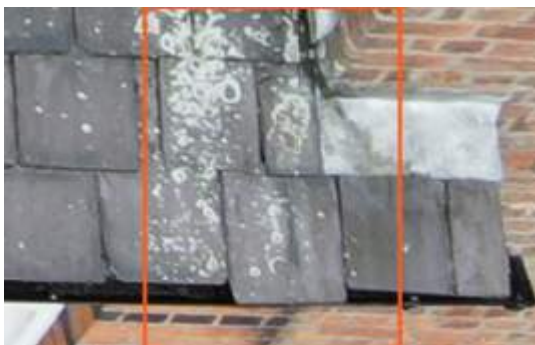
2675844 Severity: 3 Slipped Slate
