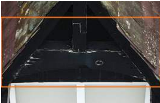
2674252 Severity: 2 Paint Coat Failed
