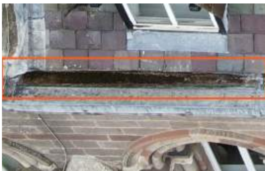
2674210 Severity: 3 Minor Debris in Gutter
