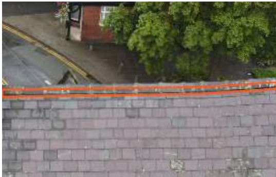
2674772 Severity: 3 Missing Mortar to Ridge
