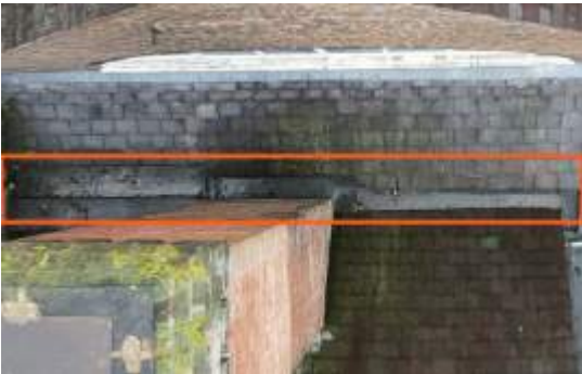
2675920 Severity: 3 Minor Debris in Gutter
