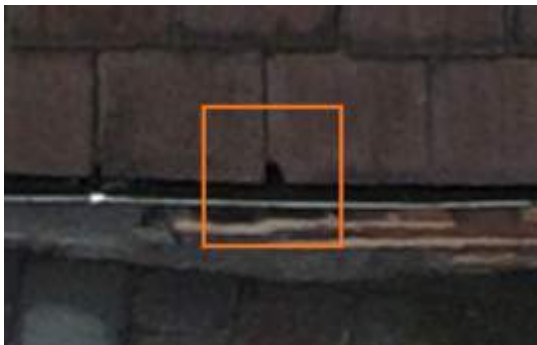
2674640 Severity: 2 Damaged Slate
