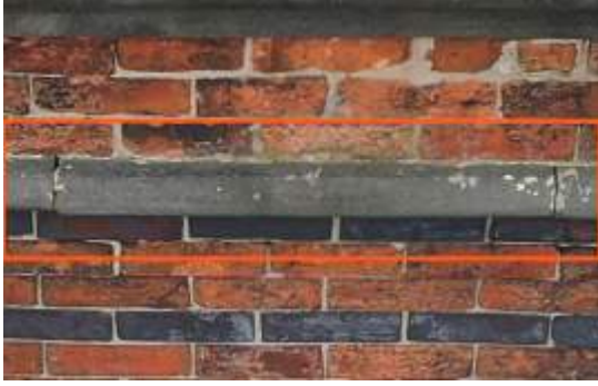
2675897 Severity: 3 Missing Mortar
