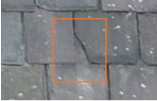
2675846 Severity: 2 Damaged Slate
