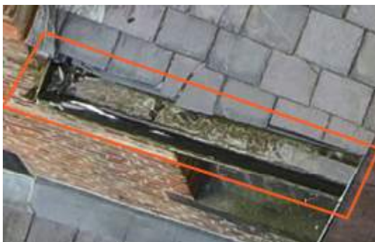
2674720 Severity: 3 Minor Debris in Gutter
