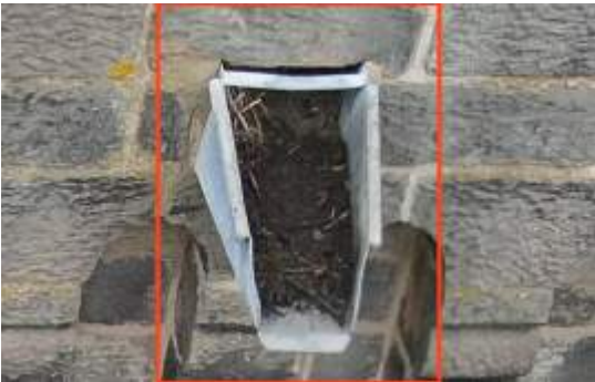
2674743 Severity: 4 Blocked outlet
