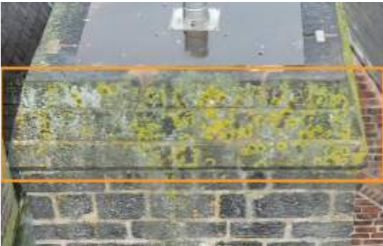
2674334 Severity: 1 Lichen Build Up
