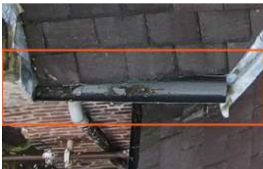
2674301 Severity: 3 Loose/Misaligned Gutter
