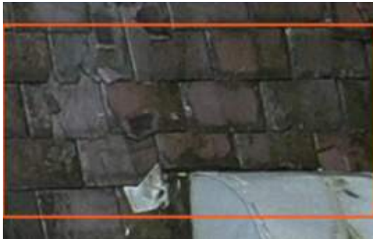
2675552 Severity: 3 Damaged Slate
