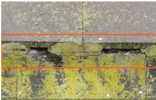
2675895 Severity: 3 Missing Mortar
