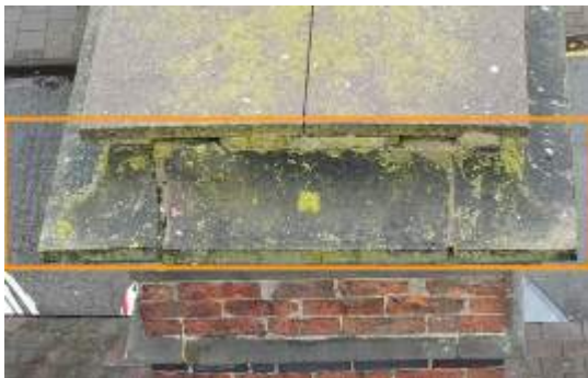
2675874 Severity: 1 Lichen Build Up
