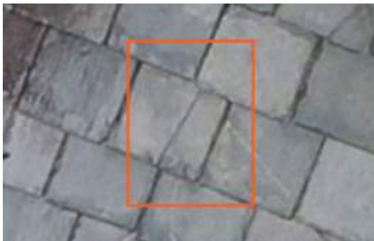
2674719 Severity: 3 Damaged Slate
