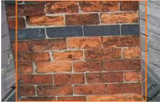
2675824 Severity: 2 Spalled Brick
