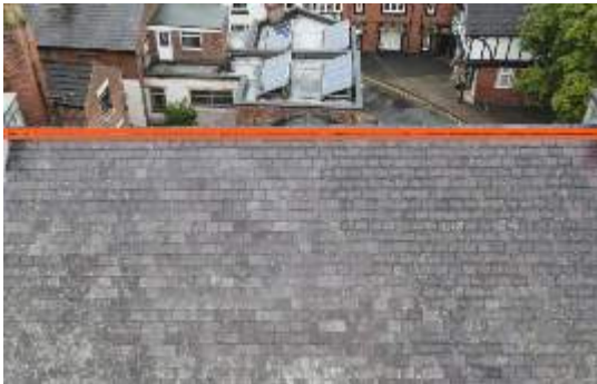
2674767 Severity: 3 Missing Mortar to Ridge
