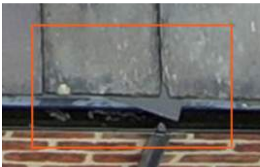
2675798 Severity: 3 Slipped Slate
