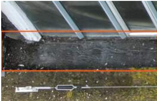
2675906 Severity: 3 Minor Debris in Gutter
