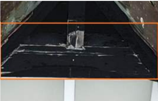
2674250 Severity: 2 Paint Coat Failed
