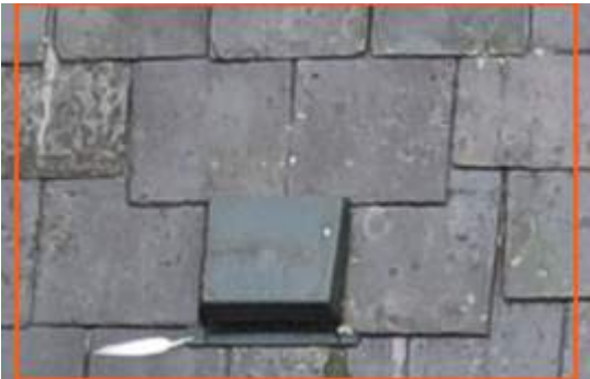
2675712 Severity: 3 Slipped Slate
