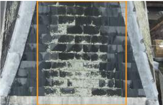
2674752 Severity: 1 Lichen Build Up
