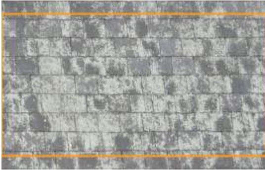
2674757 Severity: 1 Lichen Build Up
