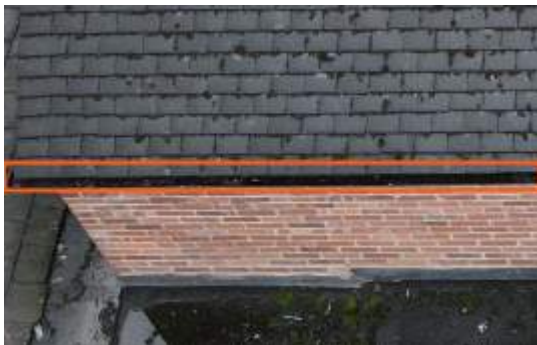
2675669 Severity: 3 Minor Debris in Gutter
