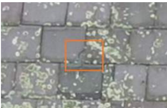
2674783 Severity: 2 Damaged Slate
