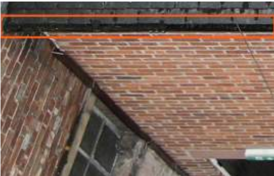
2675638 Severity: 3 Minor Debris in Gutter
