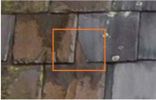
2675762 Severity: 2 Damaged Slate
