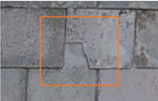
2675713 Severity: 2 Damaged Slate
