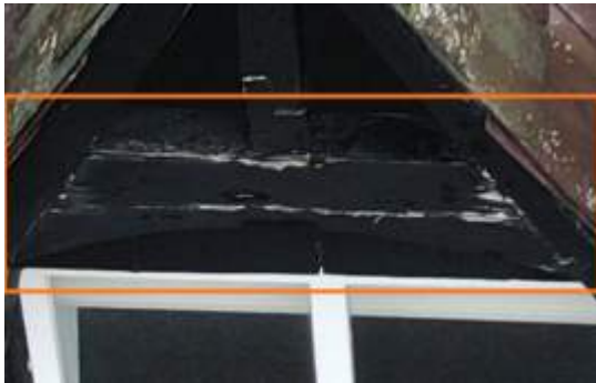
2674247 Severity: 2 Paint Coat Failed
