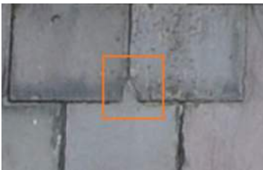
2675771 Severity: 2 Damaged Slate
