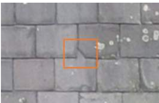
2674765 Severity: 2 Damaged Slate
