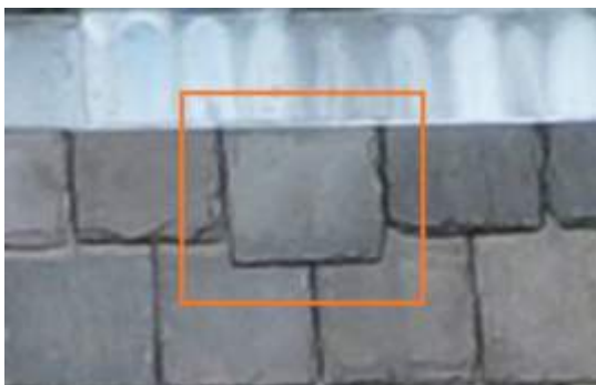
2675535 Severity: 2 Slipped Slate
