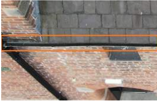
2674805 Severity: 2 Standing Water in Gutter
