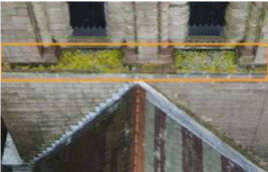
2674746 Severity: 1 Lichen Build Up
