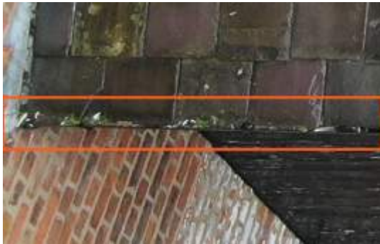
2675716 Severity: 3 Significant Debris in Gutter
