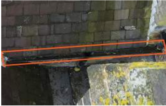
2674303 Severity: 3 Minor Debris in Gutter
