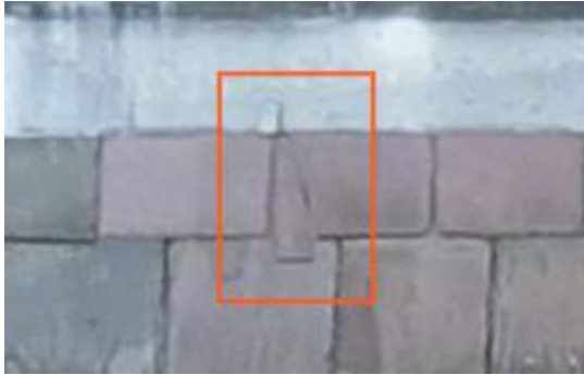
2675530 Severity: 3 Damaged Slate
