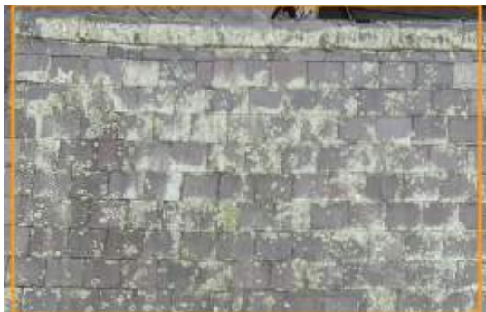
2674754 Severity: 1 Lichen Build Up
