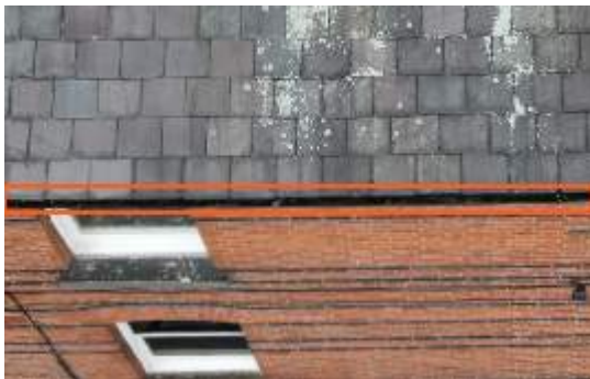
2675812 Severity: 3 Significant Debris in Gutter
