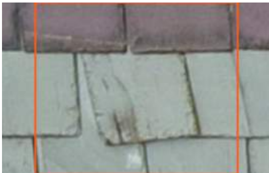
2673946 Severity: 3 Slipped Slate
