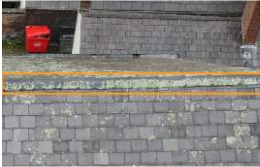
2674790 Severity: 1 Lichen Build Up
