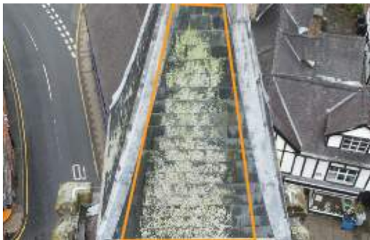
2674753 Severity: 1 Lichen Build Up
