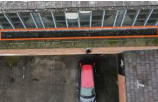
2675908 Severity: 3 Minor Debris in Gutter
