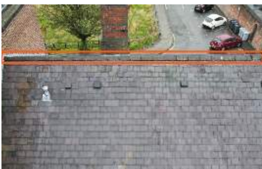
2675760 Severity: 3 Missing Mortar to Ridge
