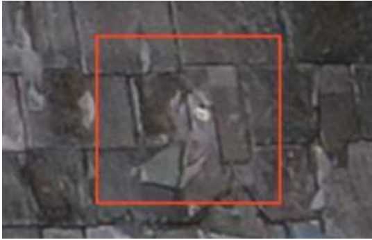
2675562 Severity: 4 Damaged Slate
