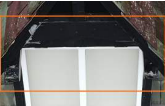
2673966 Severity: 2 Paint Coat Failed
