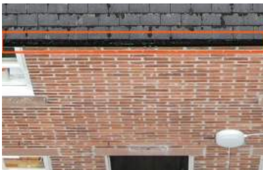
2675666 Severity: 3 Minor Debris in Gutter
