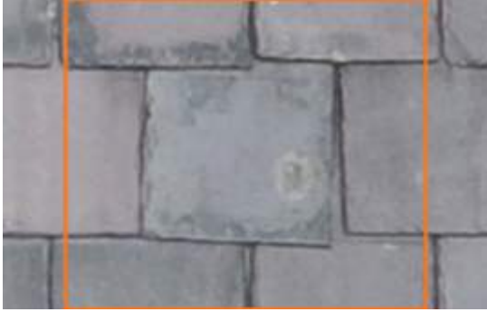
2675786 Severity: 2 Misaligned Slate
