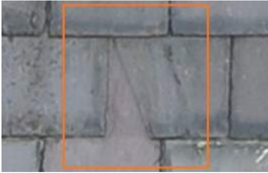
2675735 Severity: 2 Damaged Slate
