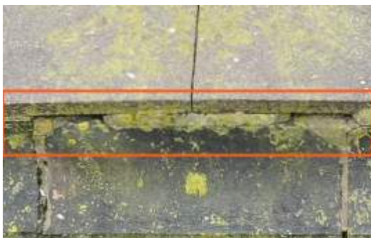
2675875 Severity: 3 Missing Mortar
