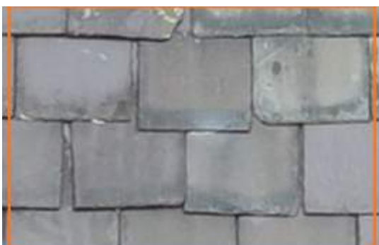
2675776 Severity: 2 Misaligned Slate
