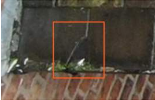
2675715 Severity: 3 Damaged Slate
