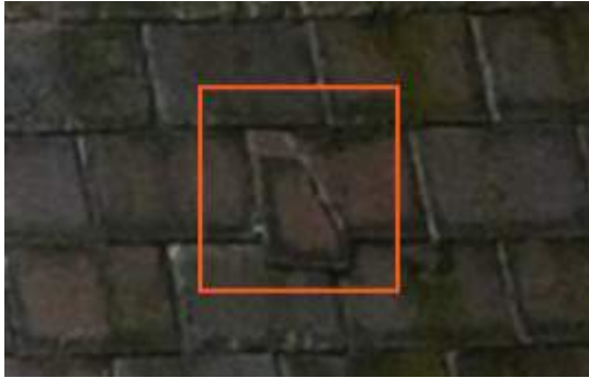
2675551 Severity: 3 Damaged Slate
