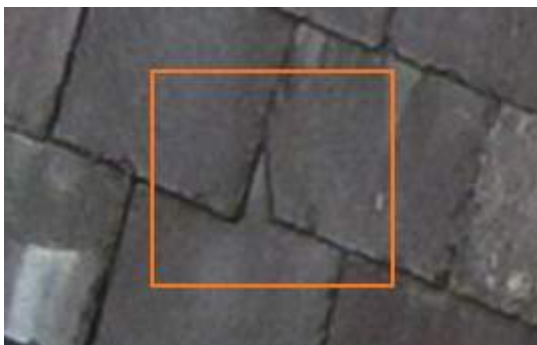
2674328 Severity: 2 Damaged Slate
