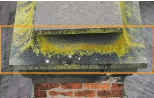
2675898 Severity: 1 Lichen Build Up
