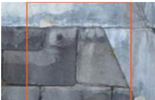
2674749 Severity: 3 Missing Slate
