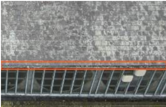
2674758 Severity: 3 Significant Debris in Gutter
