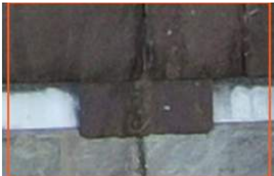
2674813 Severity: 3 Slipped Slate
