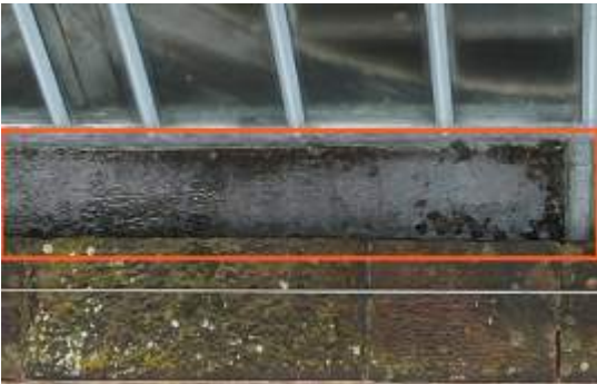
2675911 Severity: 3 Minor Debris in Gutter
