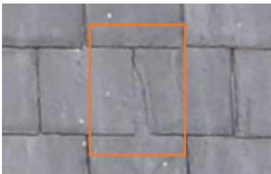
2675837 Severity: 2 Damaged Slate
