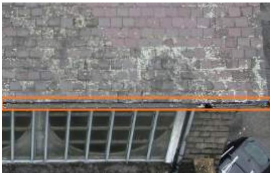
2674773 Severity: 2 Standing Water in Gutter
