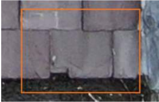
2674217 Severity: 2 Damaged Slate
