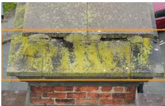
2675896 Severity: 1 Lichen Build Up
