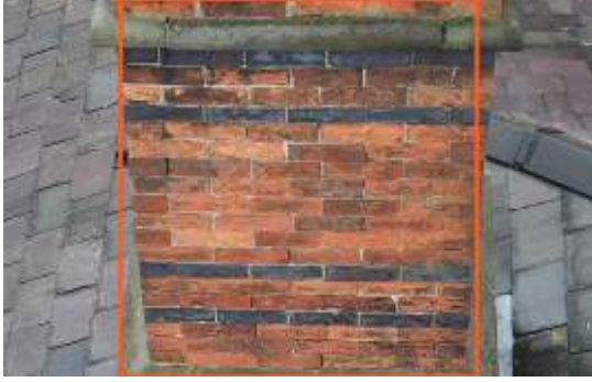
2675892 Severity: 3 Missing Mortar
