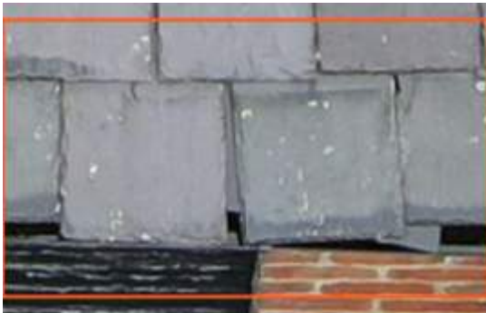
2675744 Severity: 3 Slipped Slate
