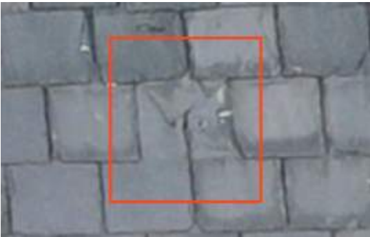
2674842 Severity: 4 Damaged Slate
