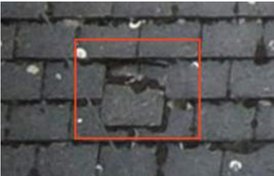
2675631 Severity: 4 Damaged Tile
