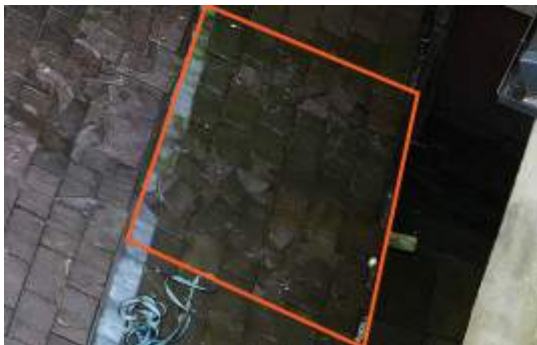
2675584 Severity: 3 Damaged Slate
