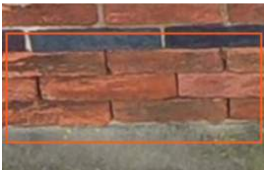
2675886 Severity: 3 Missing Mortar
