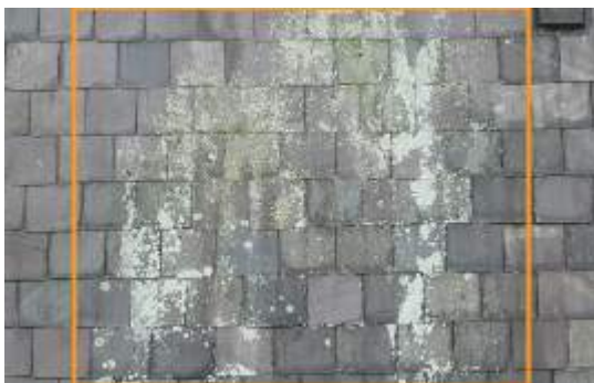
2675817 Severity: 1 Lichen Build Up
