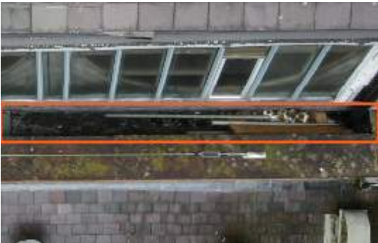
2675912 Severity: 3 Significant Debris in Gutter
