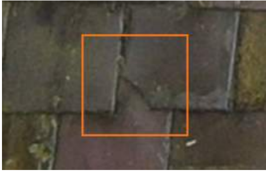
2675714 Severity: 2 Damaged Slate
