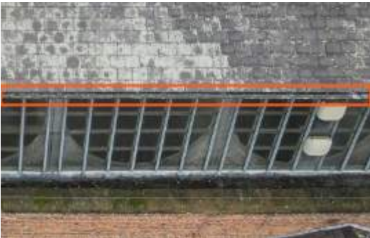
2674762 Severity: 3 Significant Debris in Gutter
