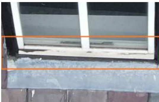
2674248 Severity: 2 Paint Coat Failed
