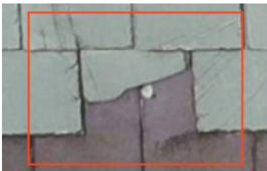
2673947 Severity: 4 Damaged Slate
