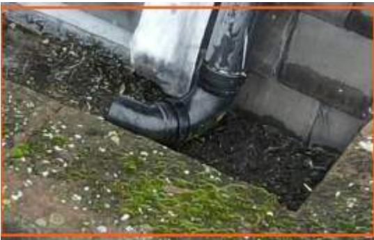
2675853 Severity: 3 Significant Debris in Gutter
