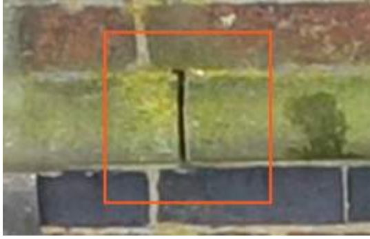
2675863 Severity: 3 Missing Mortar
