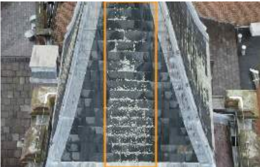
2674751 Severity: 1 Lichen Build Up
